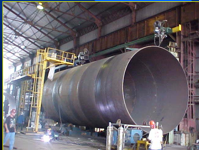
P3 Pile Section Being Welded
