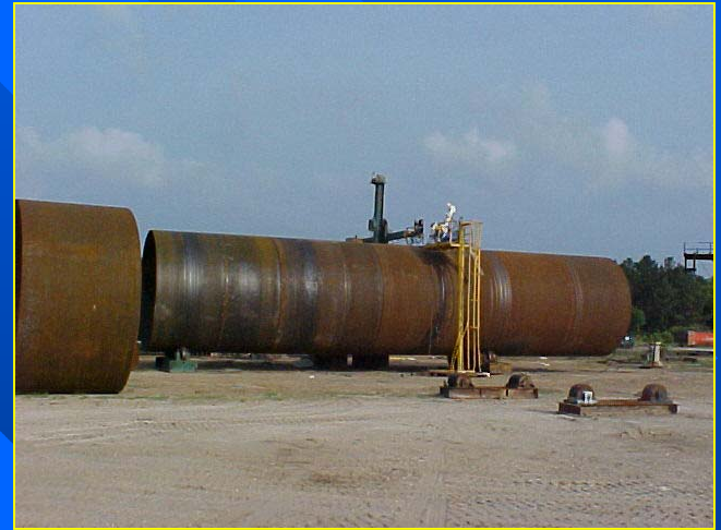
Girth Seams Being Welded
