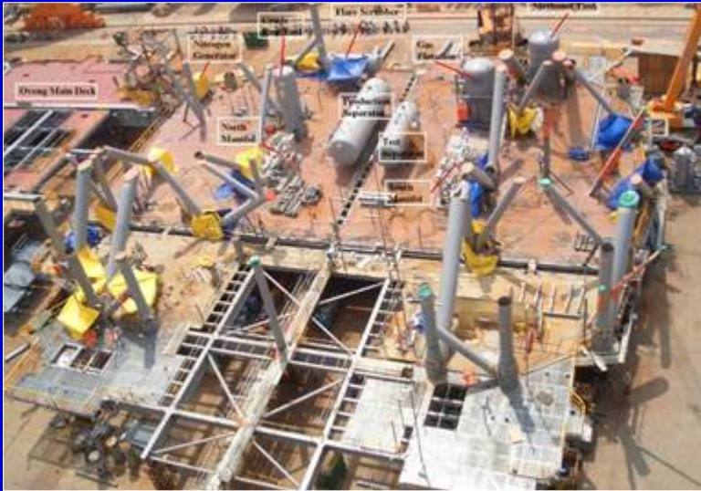
Oveng Cellar Deck
