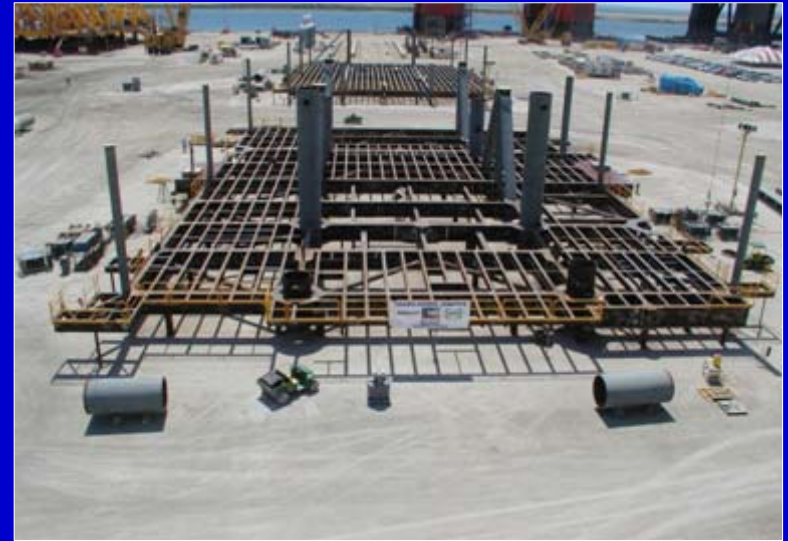
CPF cellar deck framing
