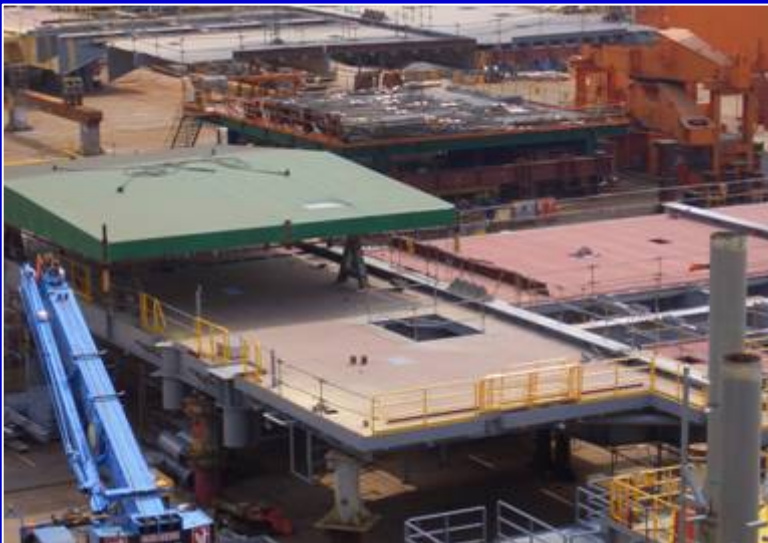
Oveng Main Deck
