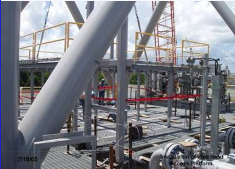
Installation of Well Head Access Platform
